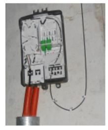
▲ Direct breakout from the ODB using Miniflex UV resistant fiber cable
